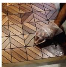
Step-9: Fill epoxy grout material
