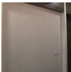
Step-1: Provide a dry & levelled wall surface
