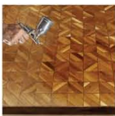
Step-8: Spray 2 coats of standard polyurethane wood sealer coatings
