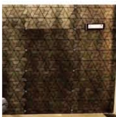
Step-6: Use spacers for interlocking panels
