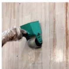
Step-4: Apply glue to liner material
